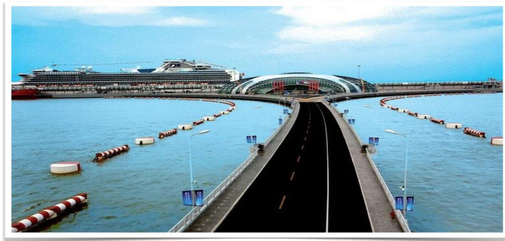
Port of Baoshan has two stops for large-sized cruise ships along its 774-meter coastline that was established during the first stage of construction, so this terminal was capable of docking a single 100,000-ton cruise ship and a single 200,000-ton cruise ship at the same time.
