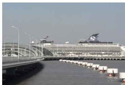
※Overall view of Wusongkou International Cruise Terminal
